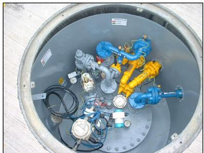
The Guide stresses the need to minimise the number of direct connections below the liquid level to lower the risk of leakage of liquid LPG. Wherever possible, only one connection, excluding the drain line, should be provided and all the rest should terminate in the vapour space.
