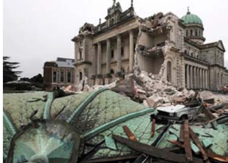
Image shows the collapsed Christchurch Cathedral, New Zealand
